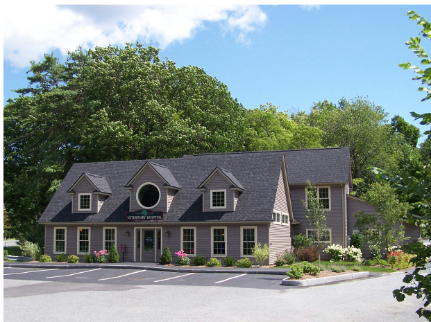
The new Stoney Brook Veterinary Hospital.
