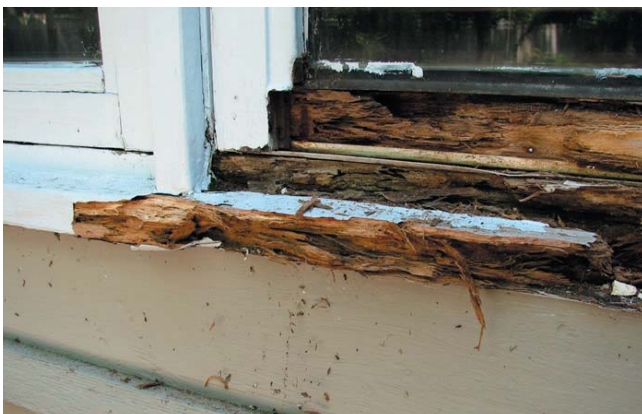
Neglected materials will decay due to weather and may require replacement that could be avoided. Historic materials and installations are preferred.
