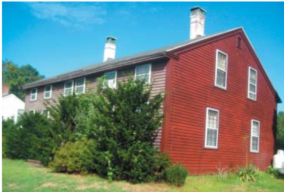
One simple gable roof is all that is necessary to shed water from this large duplex.
