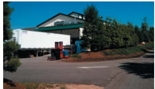
Wide entry and exit lanes, yield conditions and large curb radii allow traffic to enter or exit parking lots at dangerous speeds.
