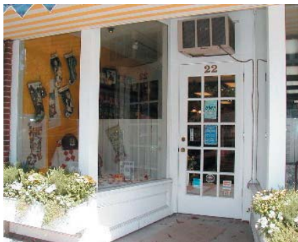
An inset entry allows more display area and a protected place to view merchandise.
