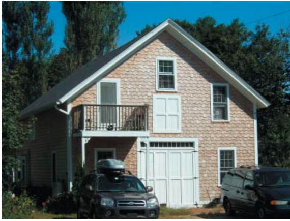
This adaptive reuse has provided a new life for a historic building that no longer serves its original purpose.
