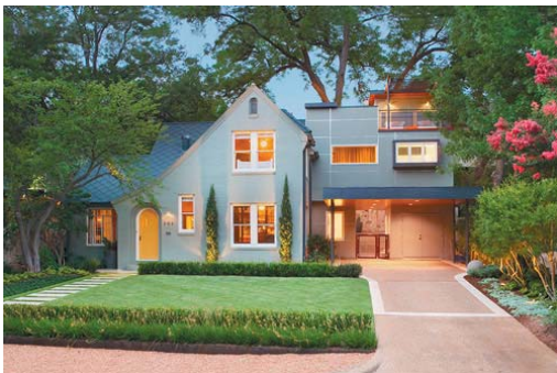
Additions that are incompatible with the existing structure destroy the character of the building.
