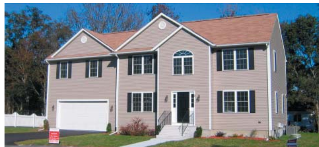
This building has been overly complicated by too many roof forms. The additional ridges, valleys and eaves are a maintenance liability.
