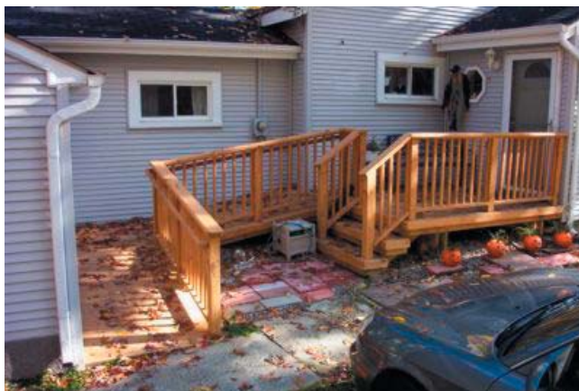
The ramp can be built of contextual materials such as this wood deck and stay close to building wall.
