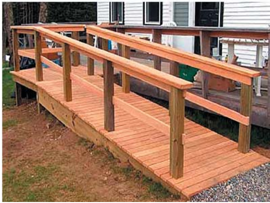
Accessible ramps where possible, should integrate with existing porches or decks and be set back from the street.
