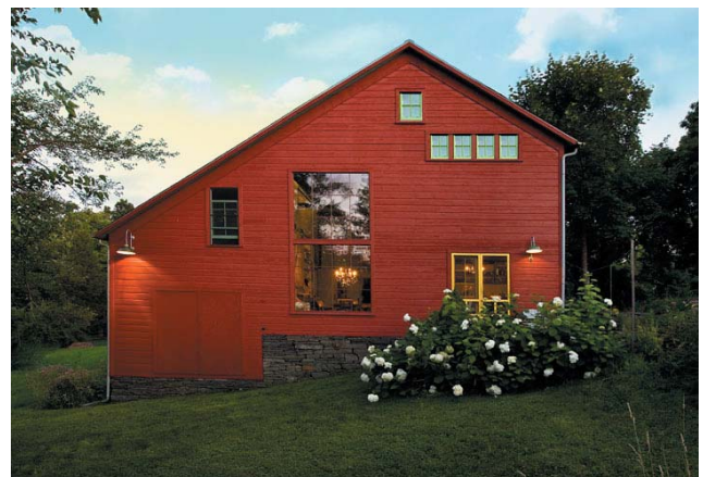
New window and door openings change the character of a converted building.
